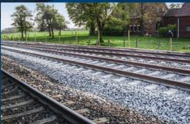
Recycled ballast consists of processed worn track ballast. It is reused as a high-quality construction material in the track bed as well as in earthworks, road and landfill construction.
