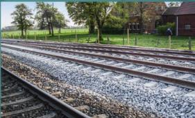
Recycled ballast consists of processed worn track ballast. It is reused as a high-quality construction material in the track bed as well as in earthworks, road and landfill construction.
